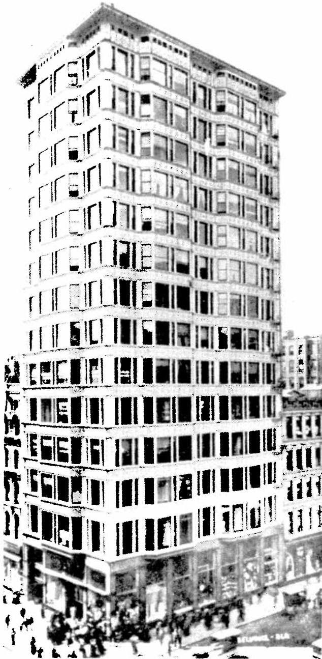
The Reliance Building represents the culmination of the development of the tall commercial structure in the late nineteenth century. The openness of its walls was emphasized by the light-colored terra cotta that covered the structural elements. The ground floor was faced with red granite, and a flat cornice topped the structure. (Photograph courtesy Municipal Reference Library)
